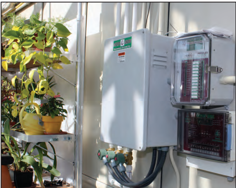
Environmental Control System in Solar Innovations, Inc.'s Greenhouse
